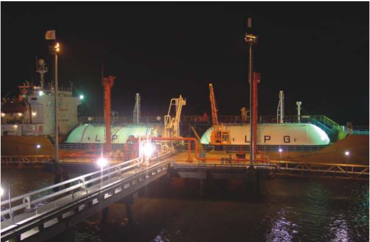
LPG cargo being off-loaded to the mass storage
