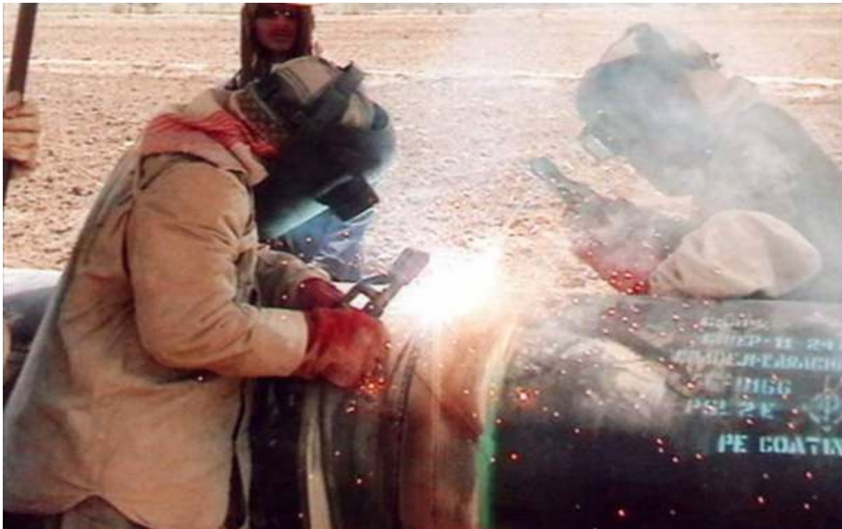
Welding Works on Main Laying
