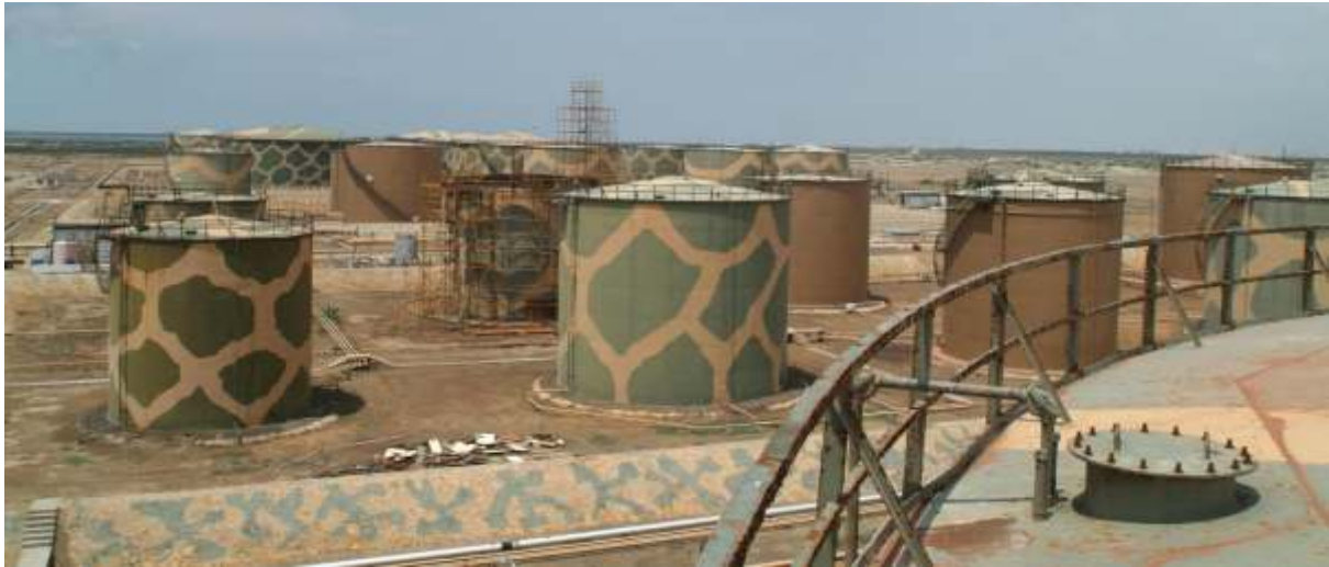
Crude Oil/Oil Products Tank Farm
