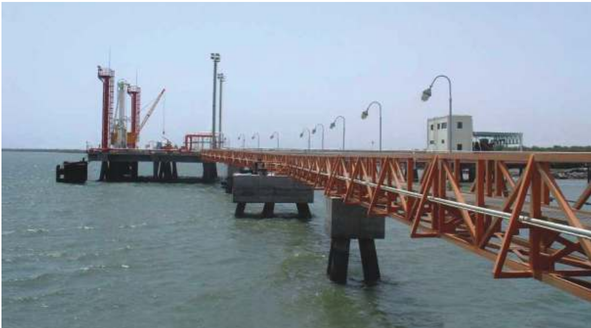
A view of the Jetty from one of the Mooring Dolphins
