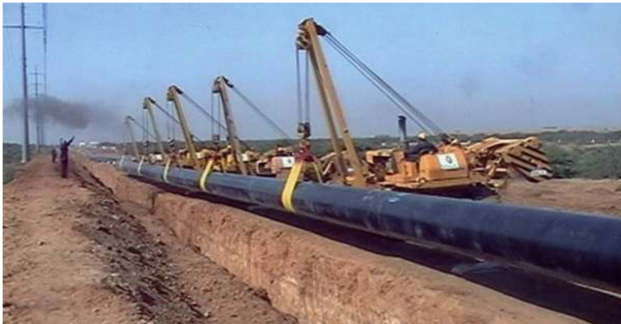
Lowering of Newly Constructed Transmission Pipelines
