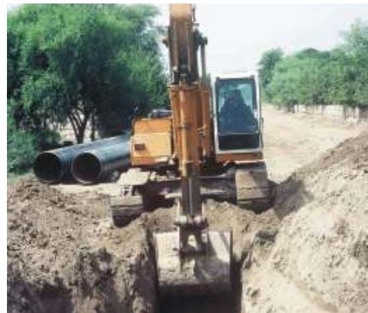
Excavation and Trenching for Laying Main Line
