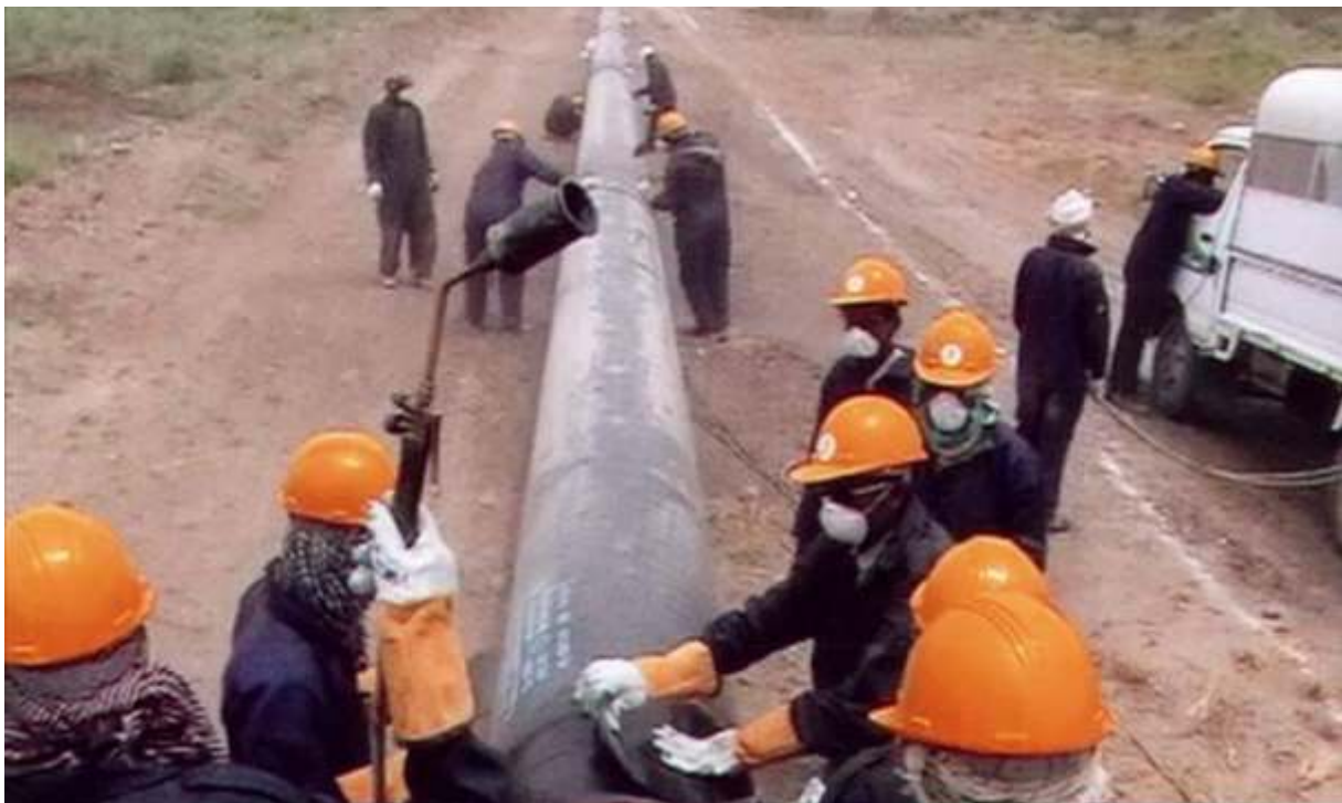
Cross Country Transmission Line being Coated
