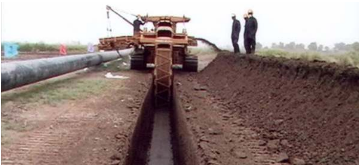
Mechanized Excavation for Main Pipe Laying
